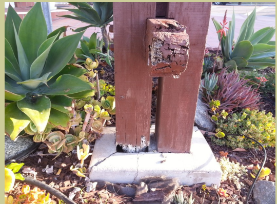
BEFORE –WOOD DAMAGE
