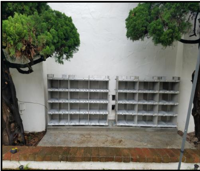
Installed open niches
